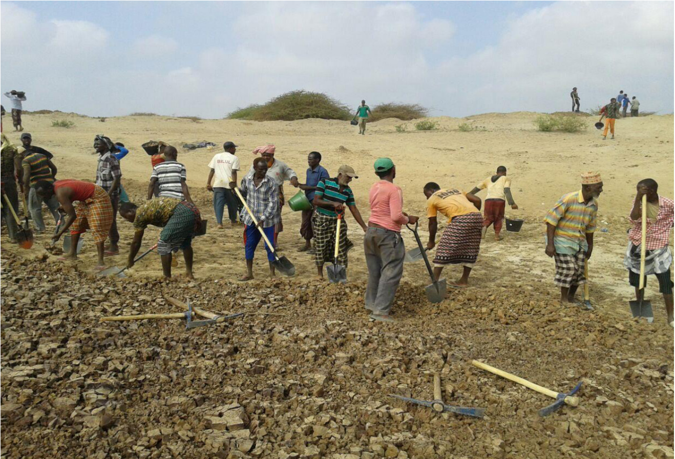
Photo 2. Community members desilting the water pan in Ras Kamboni, Somalia. Photo by ICRAF
