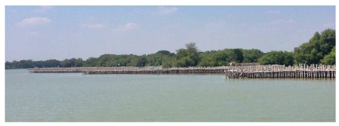
Building with Nature on the northern coastline of Java uses Hybrid engineering to rehabilitate mangroves. Local materials have been used in its construction, which enables the mangroves to trap sediment and drastically slow down erosion.
