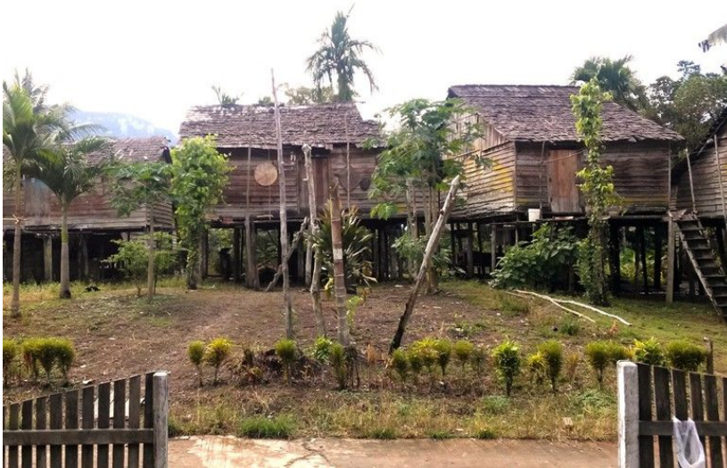
Photo 3. Houses in Rantau Bumbun Village raised on stilts for protection from floods and wild animals. Photo by Indah WB, February 2015.
