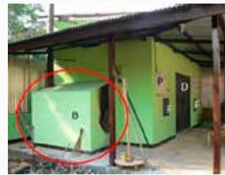
Figure 2. The completed drying chamber (A pilot project of Center for R&D FEFP2- FORDA)
