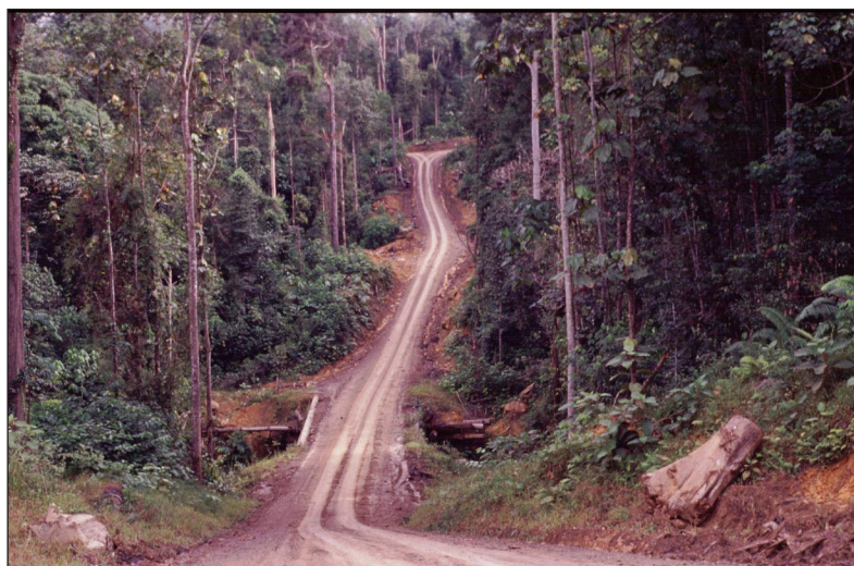
Photo 2: Well constructed road with no excessive width
