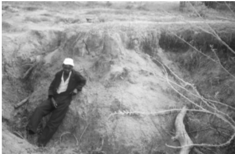
Figure 5.3 Degraded gully to be reclaimed
