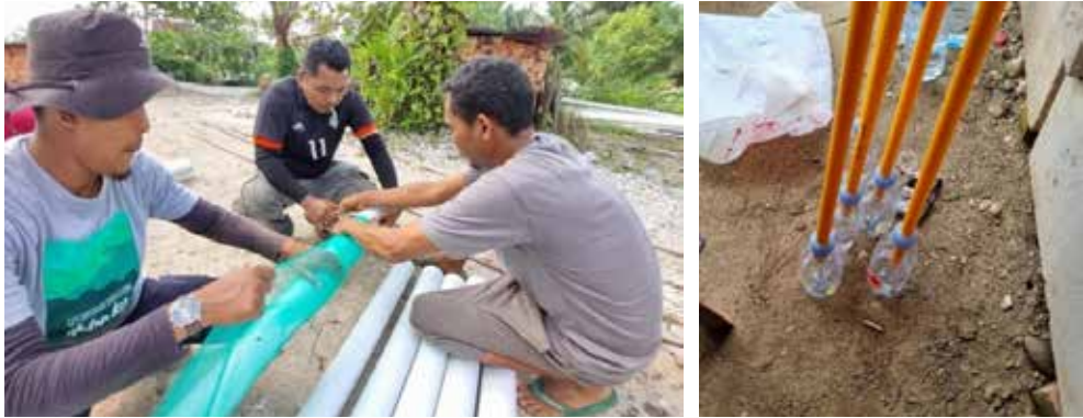
Figure 9. Dipwell pipe and floating measurement scale preparation
