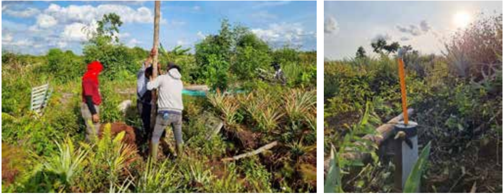
Figure 11. Installing dipwells
