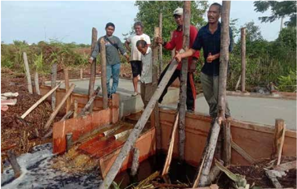
Figure 44 Canal block construction beside the main road in PGT-Action Arena 3
