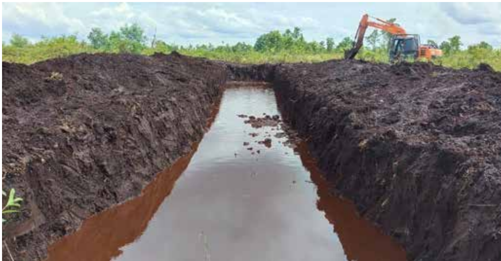
Figure 43 Pond/water reservoir construction in KAP-Action Arena 1
