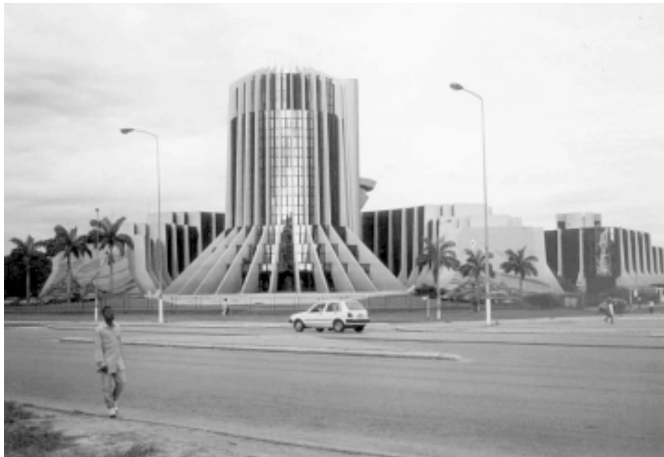
Constuction of modern government buildings in Libreville was a major item of oil-wealth spending (Photo by Sven Wunder)
