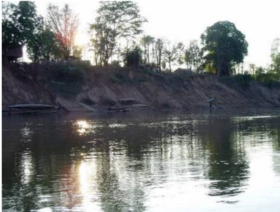
Plate 10: Sheering effect of riverbank erosion, Ban Pak Veng, February 2006.
