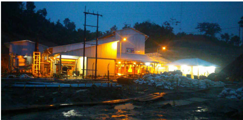
Figure 3. Documentation by CPI: The inaugural light up of the bamboo-fired power plant in Saliguma Village
