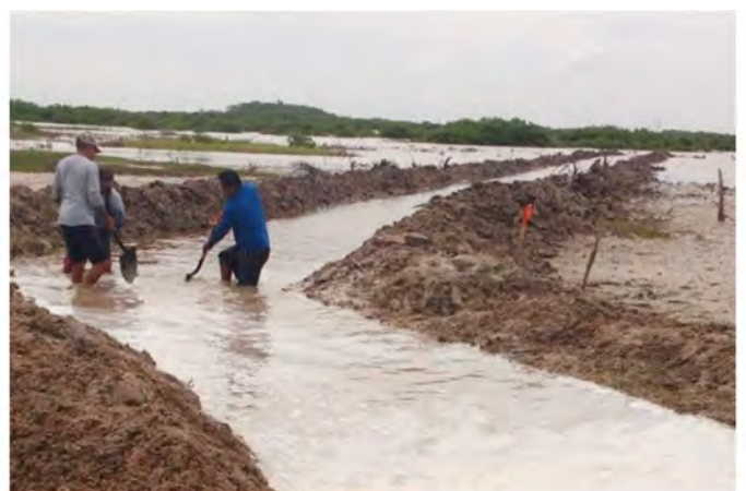
Desilting natural channels (Progreso, Yucatán).
