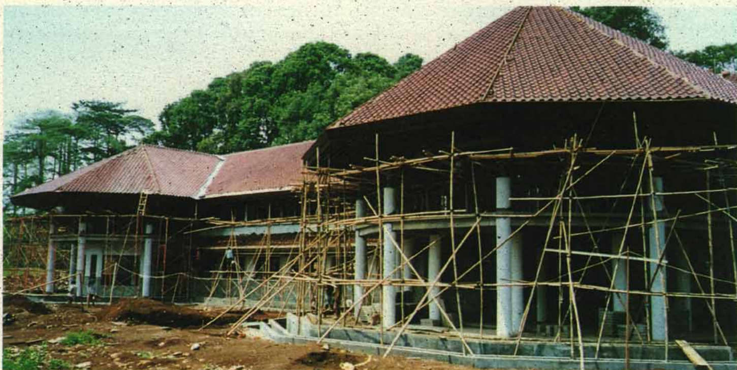
CIFOR headquarters building under construction.
