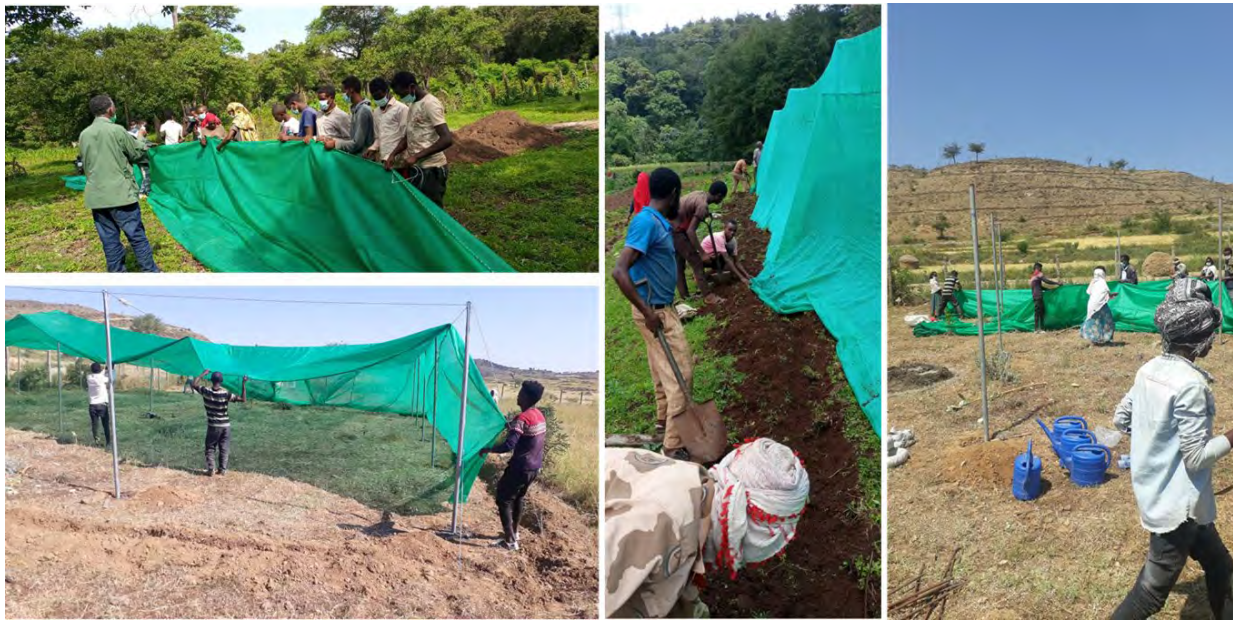
Figure 14. Building ownership through engagement in the process of establishing RRCs and nurseries: an example.
