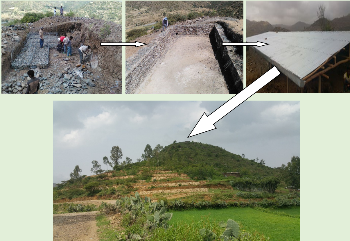
Figure 7: Partial view of piloted low-cost and innovative rainwater harvesting reservoir constructed at the top of a hill. It aims to store rainwater for irrigation of high-value trees and grasses.
