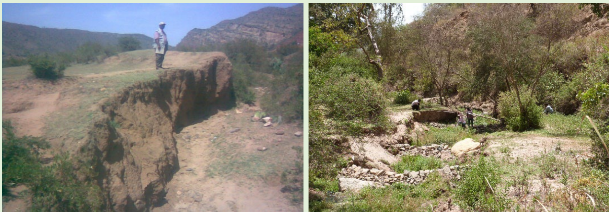
Figure 1: Partial view of scale of gullies and degradation
