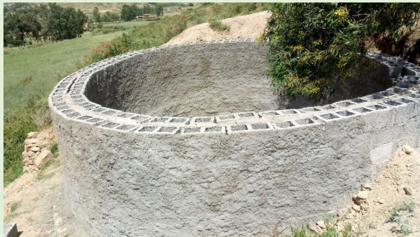
Figure 8: Partial view of road water harvesting structure. It aims to supplement rainfed agriculture and reduce runoff.
