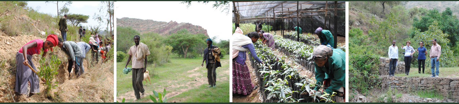
L-R: creating terraces which are then vegetated; exclosures from which local people are allowed to take only grass and leaves; production of seedlings at a Rural Resource Center to be planted out; retaining water with gabions and valley dams. Photos by CIFOR-ICRAF
