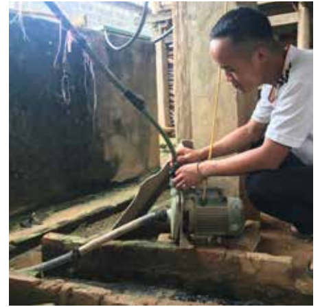
Installing pumping water system.
